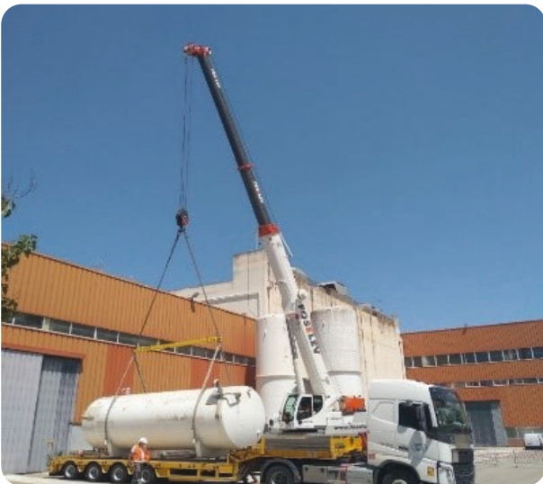
Figure 4. Loading of the 20,000l liquid helium tank for factory repair
