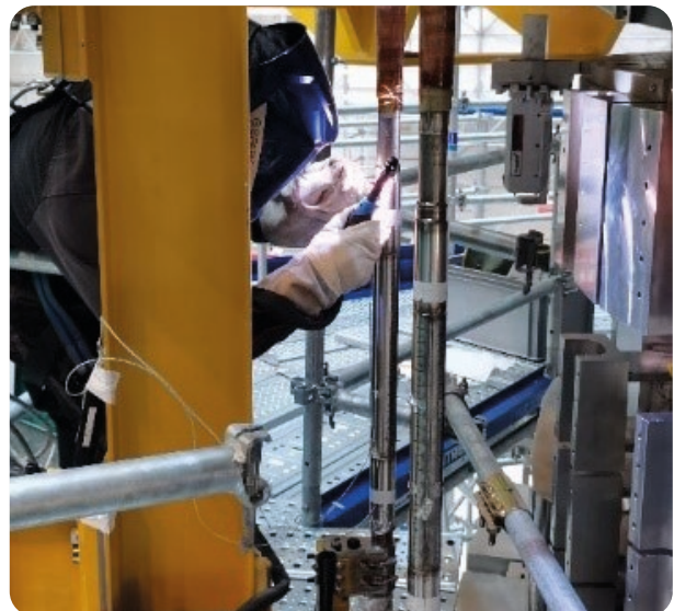
Figure 4: Production of the first superconducting joint of the central solenoid at the ITER site
