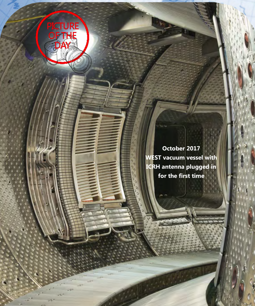
RF modelling of the WEST ICRH antenna coupling: front-face of the WEST ICRH antenna; four straps, located behind the Faraday screen, are radiating into the plasma facing the antenna.
