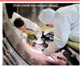
components like the Toroidal Pumped Limiter and the CFC carbon tiles of the inner bumpers were disassembled.
