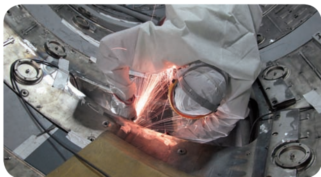
Dismantling work in the vacuum chamber
